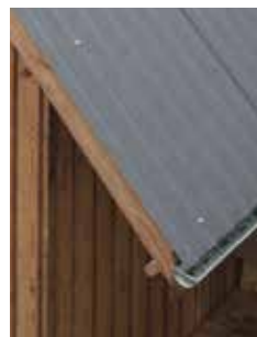
Profile corrugated metal roof sheeting
