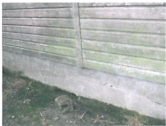
3.7 North Gable wall showing signs of deterioration at ground level.
