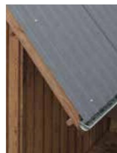
Profile corrugated metal roof sheeting
