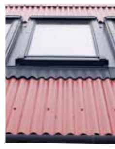
Profile corrugated metal roof sheeting
