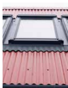
Profile corrugated metal roof sheeting
