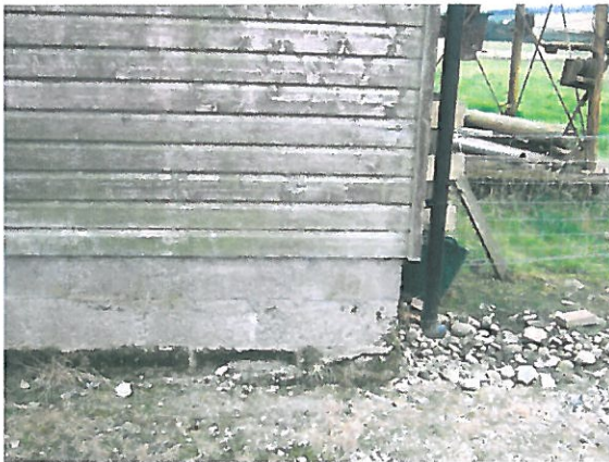
3.7 North Gable wall showing signs of deterioration at ground level.
